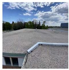
45 | 2017 | 4,990.00 | Built-up Asphalt 4ply | Good [60] | \$114,770.00 | Gravel | 26 (Yrs)
