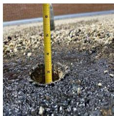
**Roof System Notes:** Two (2) test core samples were taken at the roof drain (low point, 3.5") and the roof system's perimeter (high point, 8.0").
