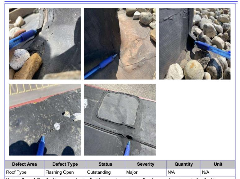
**Notes:** Open failing flashings at perimeter flashings, curb penetration flashings, and vent penetration flashings.
