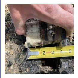
**Roof System Notes:** Two (2) test core samples were taken at the roof drain (low point, 4.5") and the roof system's perimeter (high point, 4.5").
