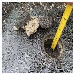
**Roof System Notes:** Two (2) test core samples were taken at the roof drain (low point, 2.0") and the roof system's perimeter (high point, 7.5").
